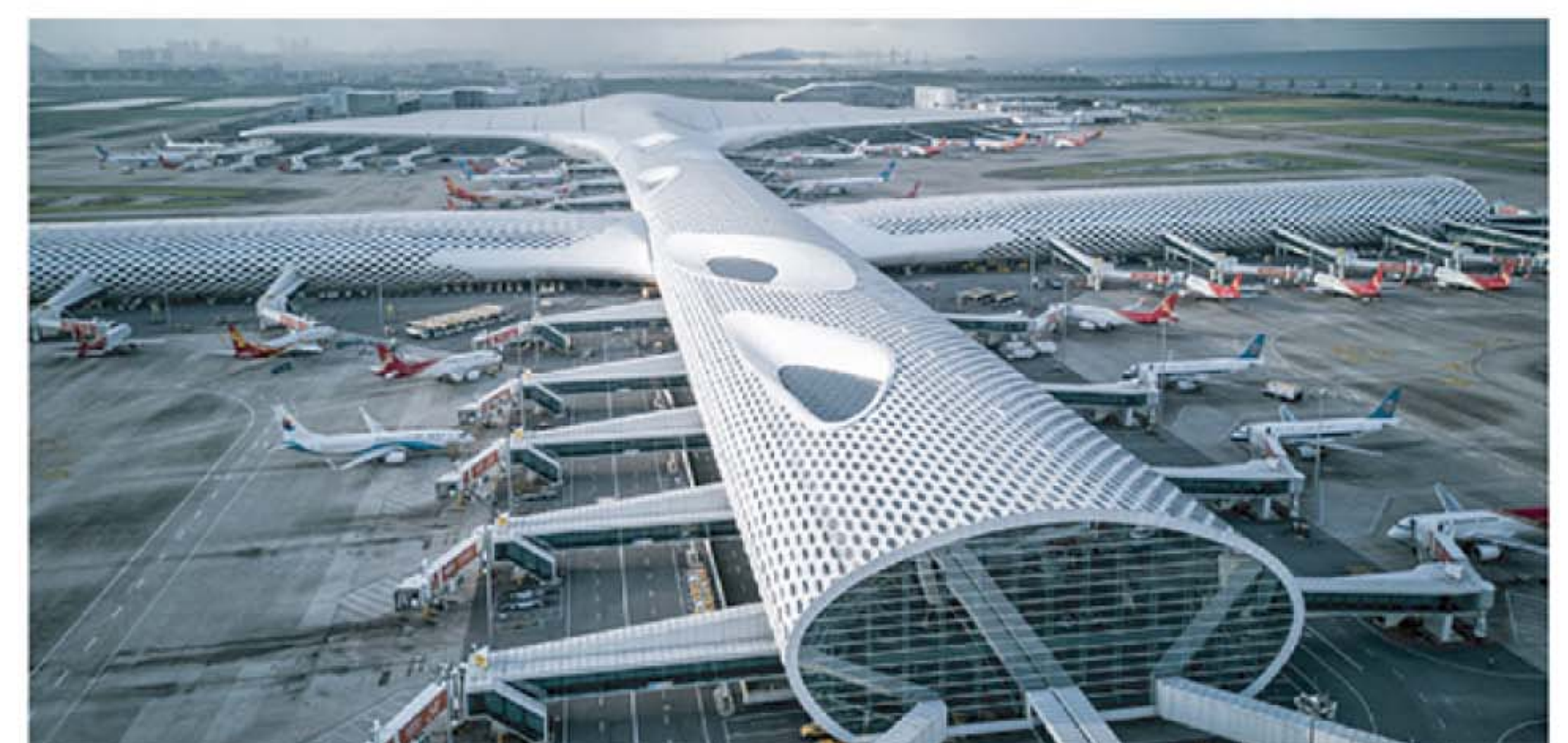
Shenzhen Bao'an International Airport Satellite Hall
